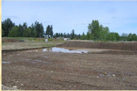
Step 1. Bring in lots of gravel to cover up high water table areas
